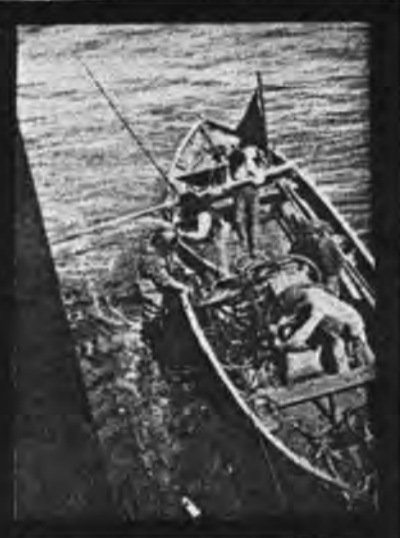
Diver repairing leak on the S.S. COYOTE.
